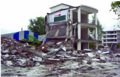
图9 局部加强后的楼梯间并未倒塌(聚源中学) Fig. 9 Stairwells local strengthened did not collapse (Juyuan Middle School)
